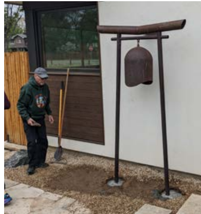
Fred Becker sets the concrete for our new temple bell.
